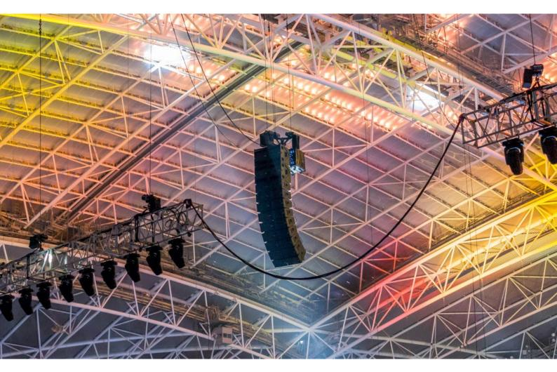
The Show Company had to work with the existing acoustic challenges because of the structural issues of the stadium especially its domeshape roof, and there was no quick solution to this. The team used NEXO's NS-1 proprietary software design and modeling software to achieve precise positioning and an optimum result, as NEXO's Nicolas Kirsch confirmed, "the sound is clear and detailed even though that huge dome shaped roof gives a 7 sec reverb time. STM is soooo precise."
