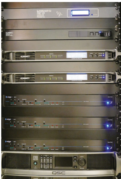
Room-combining functionality in the Western function rooms is entrusted to a Q-Sys Core 110f processor
