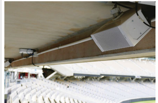
200 Nexo ID24 cabinets have been installed into the shadow areas below the L1, L3 and L4 balconies
