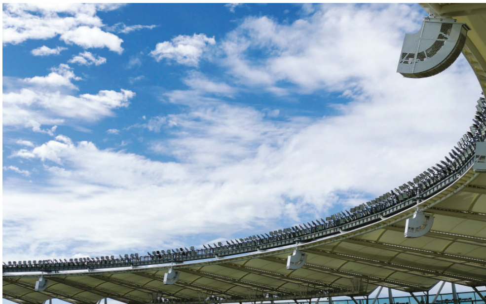
18 Nexo Geo S12 arrays suspended from the lip of the 53m-high roof provide 104dB SPL contributing to an STi of 0.6
