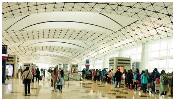
All speakers needed to be concealed behind the perforated triangular ceiling panels
