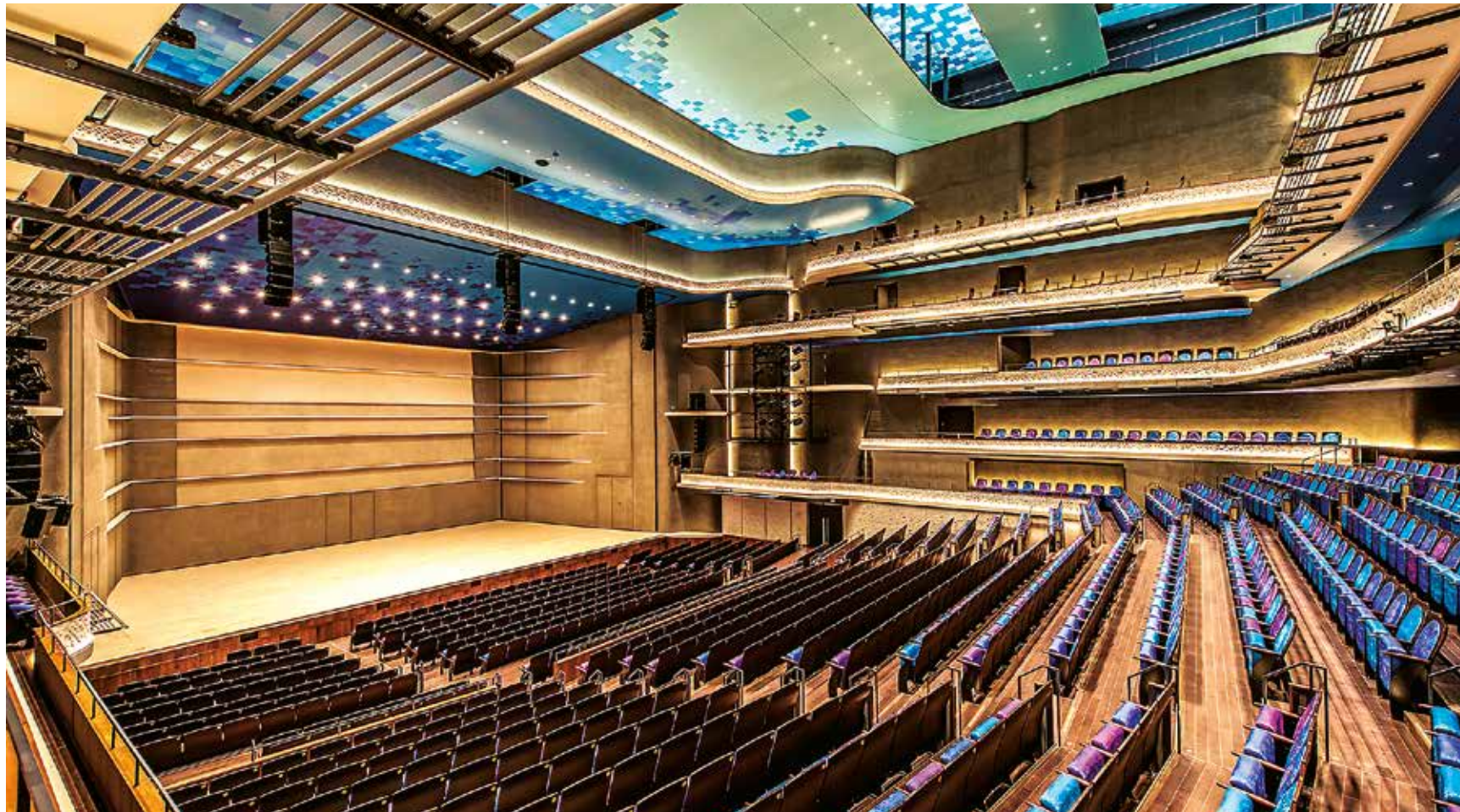
The Naha Cultural Arts Theatre on the island of Okinawa, Japan, features GEO M10 line arrays with MSUB15 subs flown LCR above the stage with additional L-R clusters and ID24s as under-balcony auxiliary speakers
